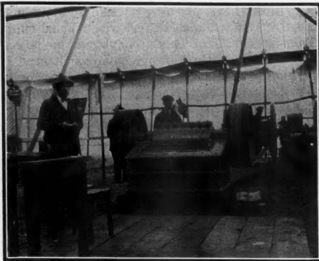
Cedar Rapids Crusher in Operation
